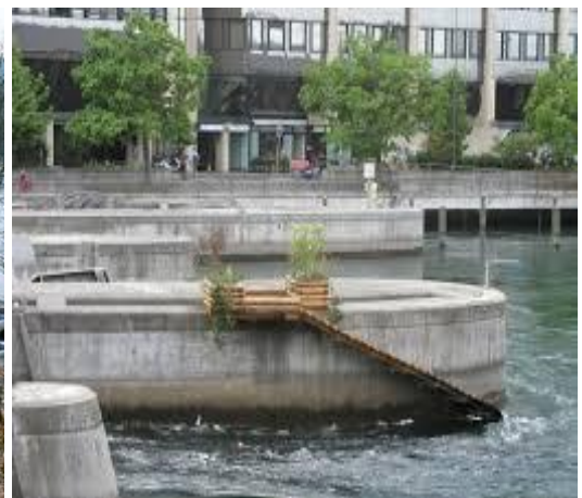
Wooden ramp for beavers at Seujet dam.
